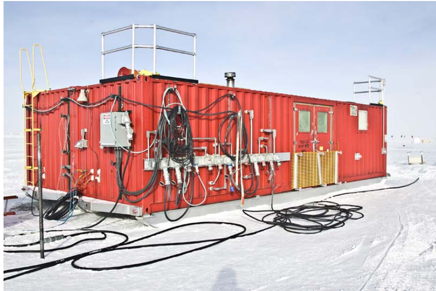
Figure 2. TOS1 and TOS2 are identical containers. Both are double-wide ISO containers, 34 feet long. On each, the power is fed to the electric heaters through a 100A Appleton connector mounted on the outside of container (gray enclosure in image). End doors are on the far end of the building, not shown.
