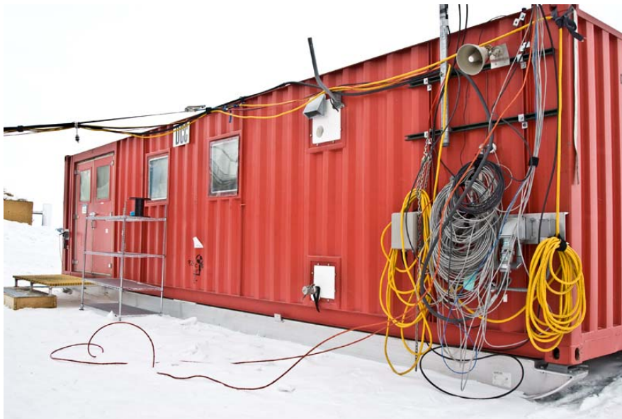
Figure 1. The DCC is a single ISO container, 34 feet long. The power is fed to the electric heaters through a 60A Appleton connector mounted on the outside of the container (shown on far right of image).
