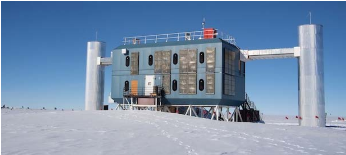
Figure 3.2-1. IceCube Laboratory (ICL). The ICL at the South Pole houses the online computing system that is critical to collecting, storing, and filtering data from IceCube.
