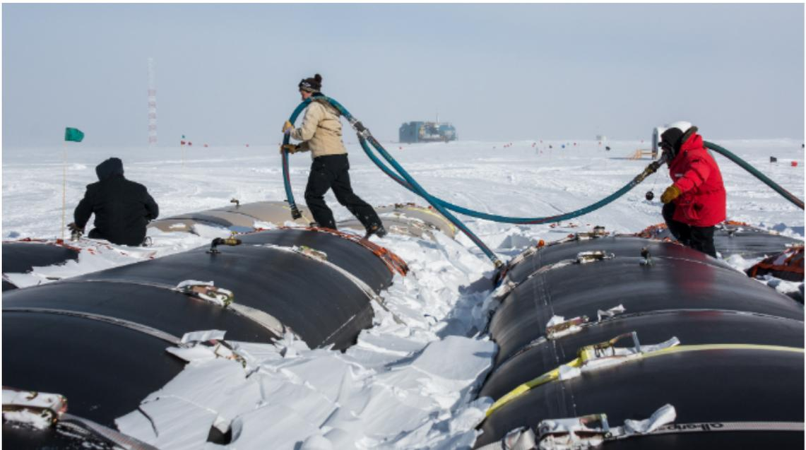
Figure 5: SPOT offloading bladder-set at Amundsen-Scott South Pole Station from [https://photolibrary.usap.gov/PhotoDetails.aspx?filename=Fuels\\_South\\_Pole\\_Hose\\_Bladder\\_transfer.jpg](https://photolibrary.usap.gov/PhotoDetails.aspx?filename=Fuels_South_Pole_Hose_Bladder_transfer.jpg)
