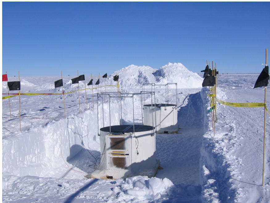
Figure 3.11: Two IceTop tanks pictured during deployment. The IceTop tanks are placed in a trench, which is filled in after deployment so that the top of each tank is level with the surrounding surface.
