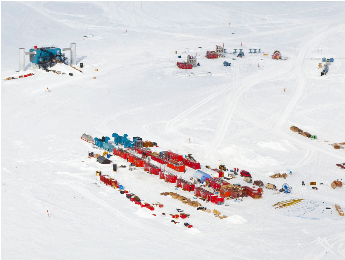
Figure 1: IceCube drill with the main heating plant in the front (seasonal equipment site), the two drill towers and the IceCube laboratory.
